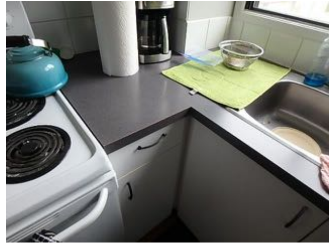
Kitchen Counter tops in some units appeared to be upgraded
