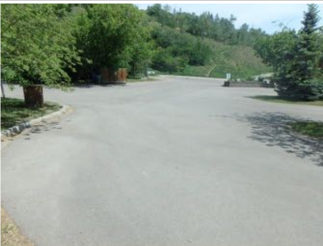
Typical Asphalt condition of main drive lane 6.
