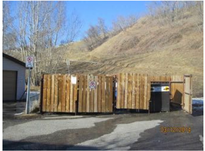
Garbage bin enclosure at the North end of Block 4 observed.
