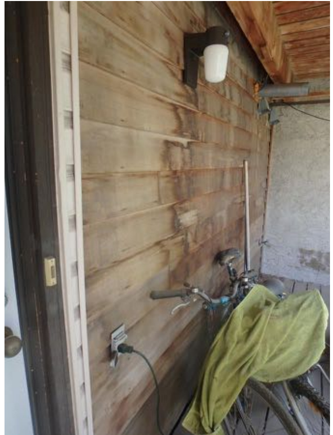
Close up view of exposed original cedar siding found on Block 1.
