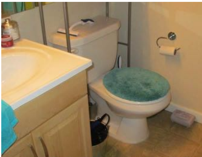
Typical standard flush toilet observed.
