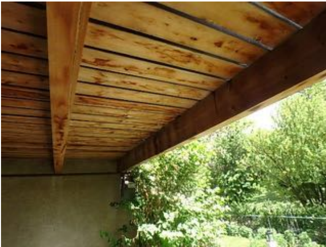
Typical close up view of the balcony wooden planks & joist underside.
