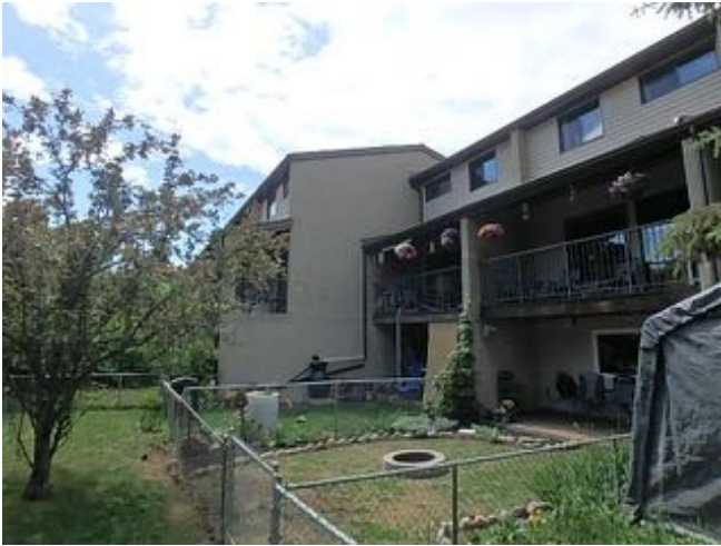
Chain link fencing & gate forming the back yard.
