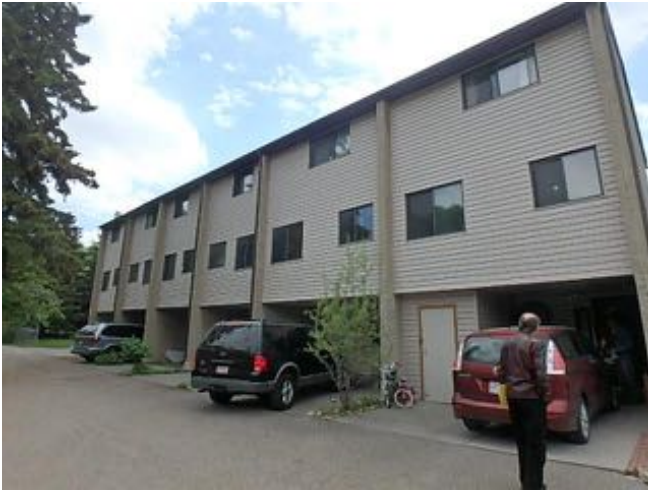
Typical siding configuration / Condition.
