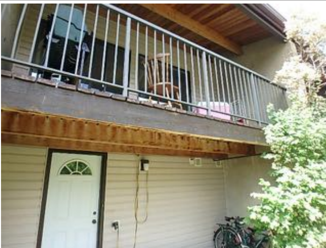
Typical replaced rear entrance door.
