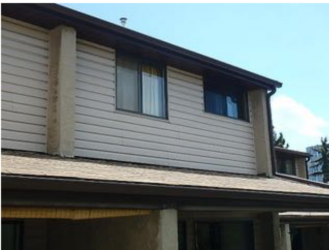
Typical Asphalt condition over balcony areas
