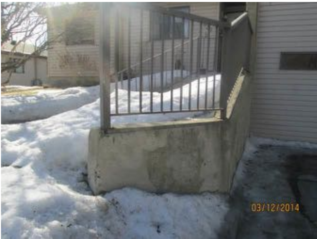
Concrete retaining wall with metal guardrails at Block 6.
