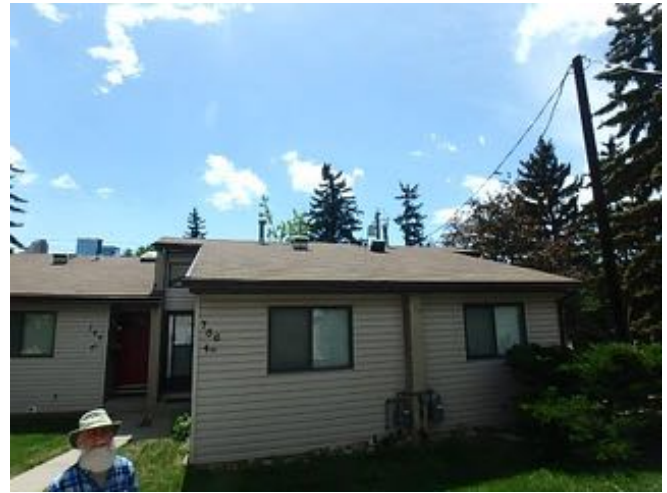
Typical Asphalt roof condition on single storey units.
