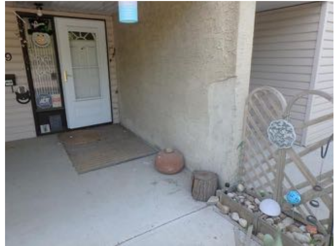
Enhanced Front Entrance Door with Screen Door and Side lite
