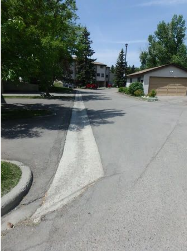
Overview of asphalt paving adjacent Common Garage.
