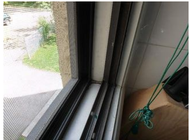
Typical sliding window track configuration and condition..
