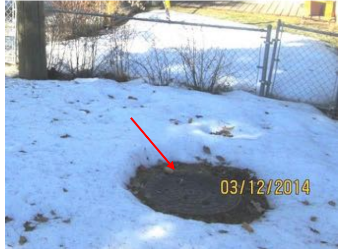
Typical catch basin to storm sewer system observed near Block 4.
