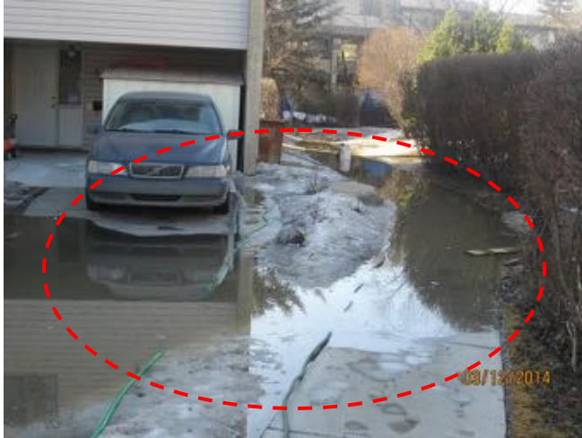
Ponding water observed at the driveway & concrete walkway between Blocks 1 & 2.
