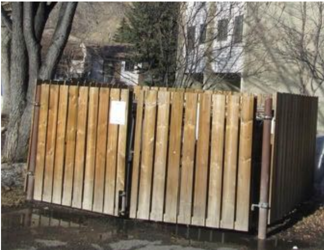
Garbage bin enclosure near Block 3.
