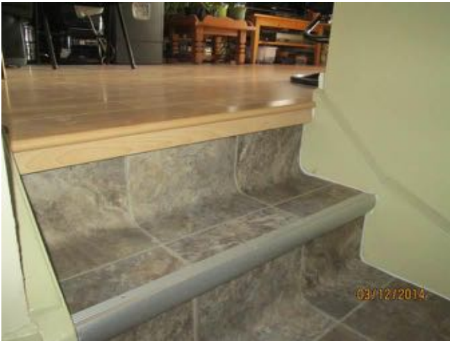
Typical recently upgraded flooring in a townhouse unit.
