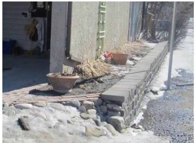
Interlocking block retaining wall around planters at Block 8 observed.
