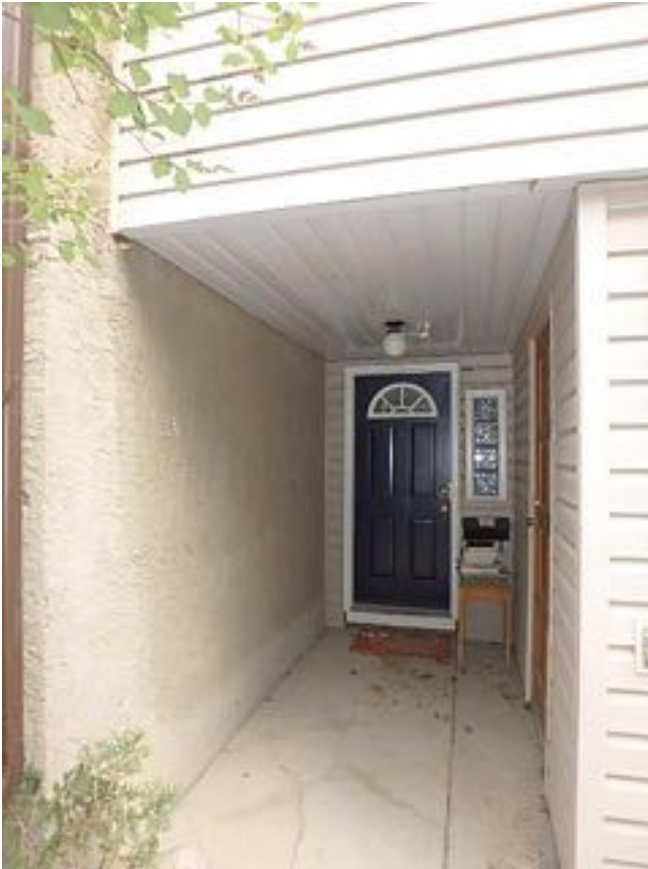
Typical townhouse unit main entrance door.
