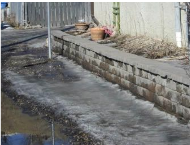
Retaining wall around planter at West end of Block 8 observed.
