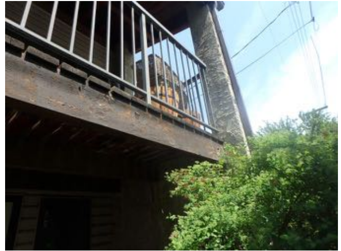
View of weather finishes on deck joist
