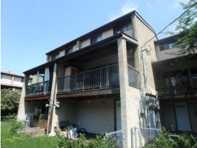
Typical fascias, soffits, eaves troughs and downspouts.
