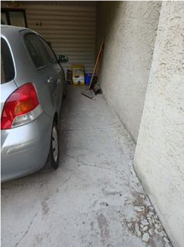
Typical concrete slab at the carport.
