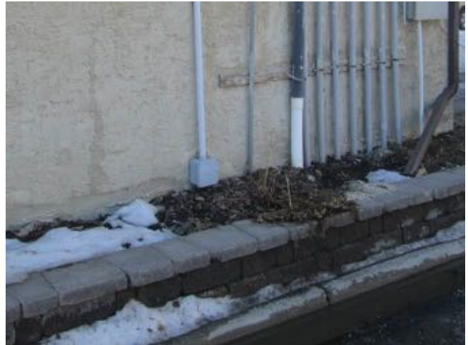
Interlocking block retaining wall around planters at Block 4 observed.
