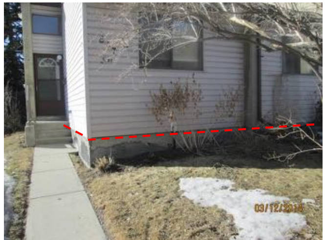
Typical foundation walls of a townhouse unit reviewed.
