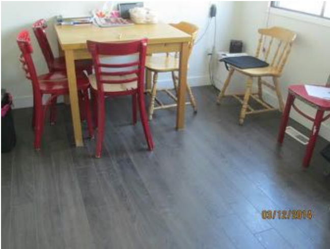
New laminate flooring observed in multiple units reviewed.
