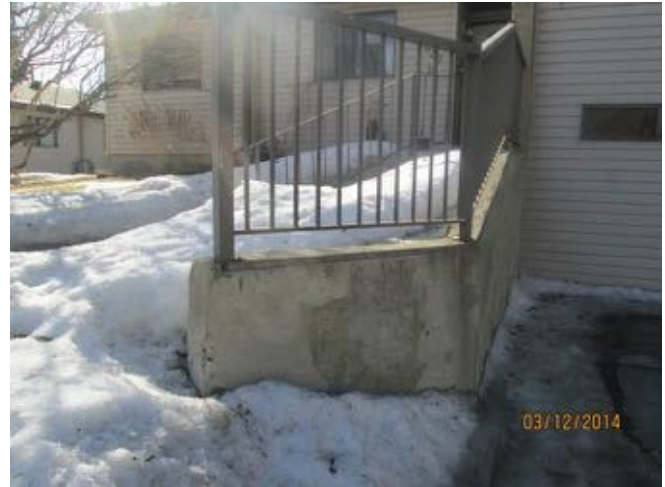
Typical metal guardrail on top retaining wall at Block 6 observed.
