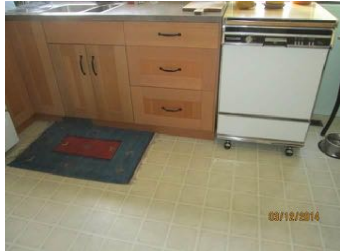
Vinyl sheet flooring in the kitchen of a unit observed.
