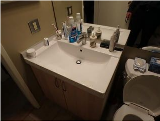
Recently upgraded bathroom components included newer counter top and faucet
