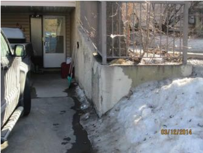
Concrete retaining walls at Block 4 between townhouse units.
