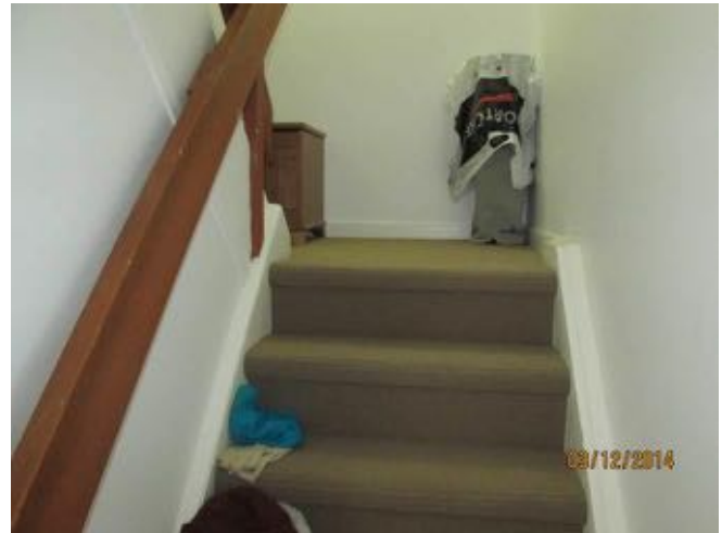
Carpet flooring observed in the unit's staircase at Block 6.
