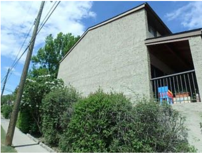
Typical low to moderately sloped roof area.
