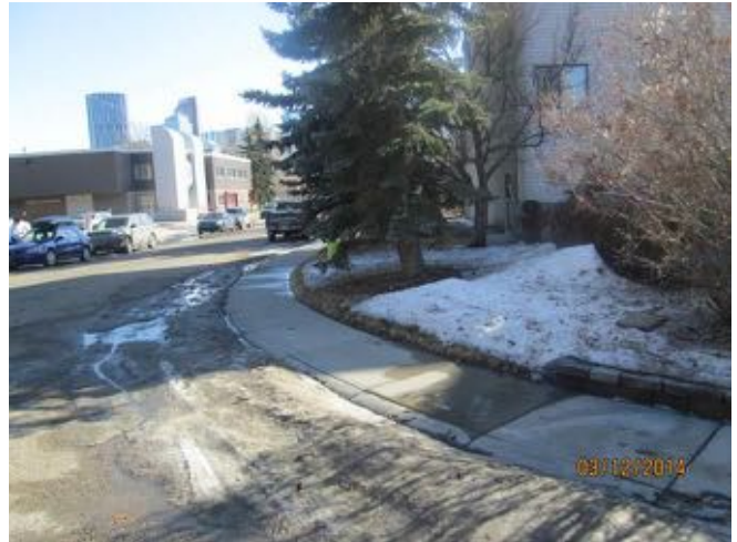
Typical concrete walkways & curbs near Block 2 observed.
