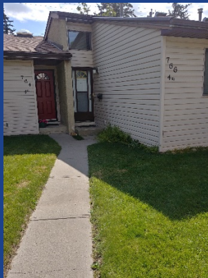
Figure 4: Entry doors with steps
