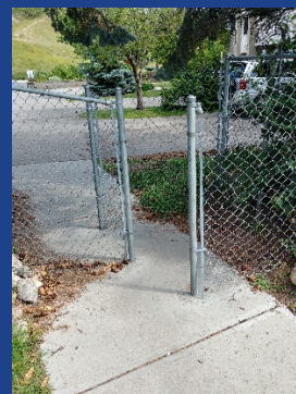
Figure 3: Maze entrance at rear gate
