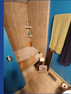
Figure 8: Tubs require high step to enter and most have no grab bars.
